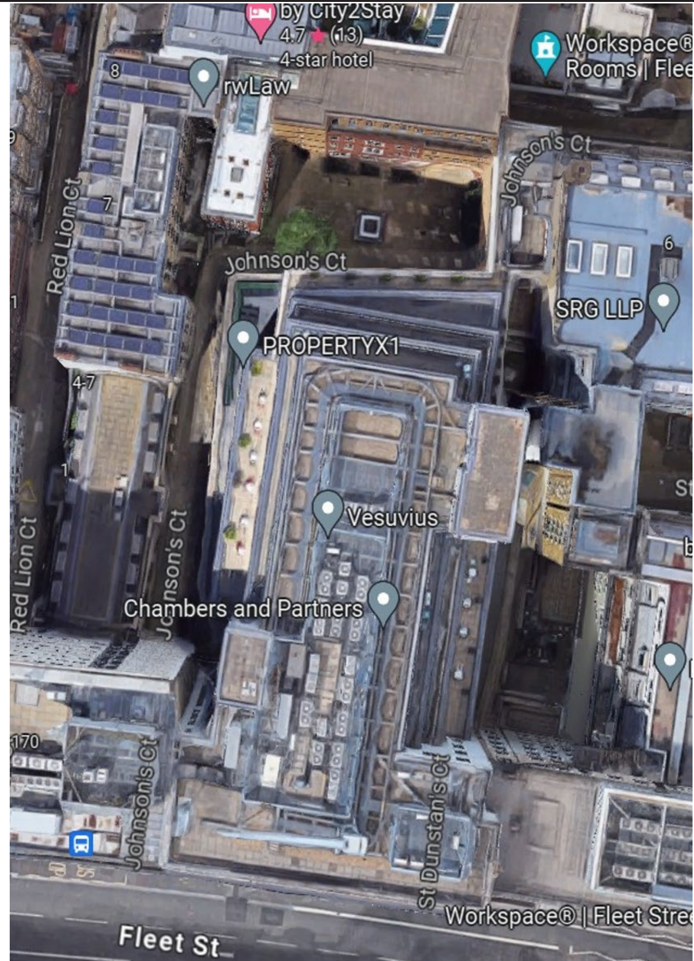
Existing Building – aerial view
