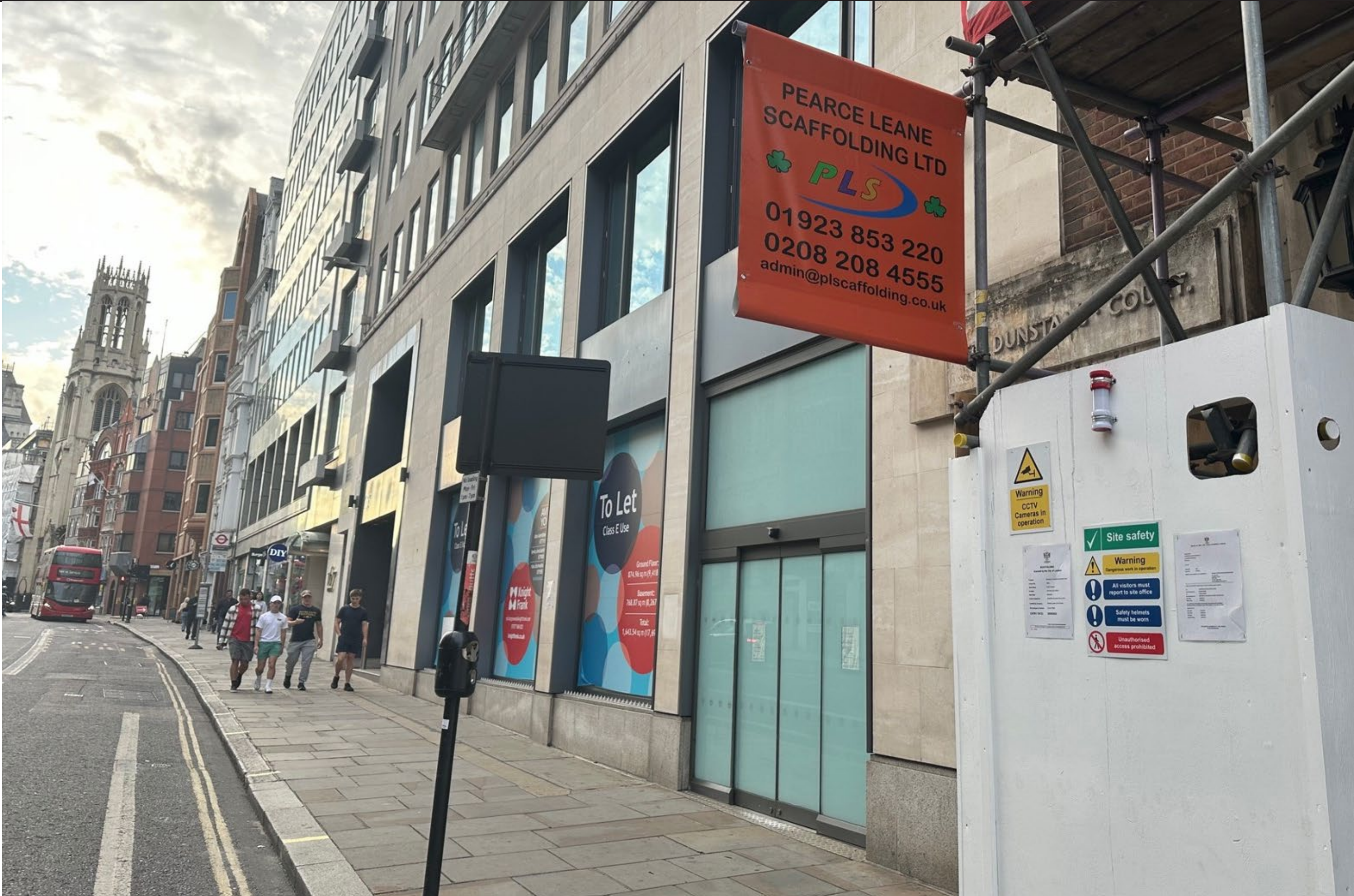
Existing Unit – Fleet Street View West
